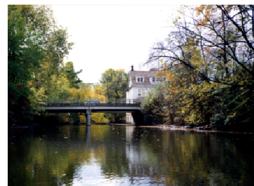
River Edge Road bridge between River Edge and New Milford
