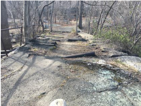
Bear Swamp Dam - Does This Look Safe to You?
